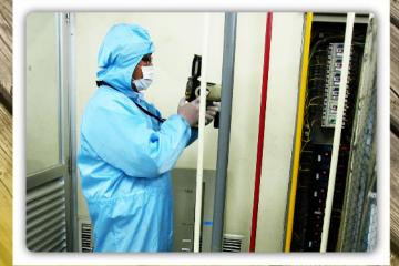
With the commitment of RT Asurans. Tokks Marine Indonesia to become one of the best general insurance companies, as a value-added service we offer an infrared survey assistance to our corporate customers. The infrared survey has the ability to detect a surface temperature of a particular inspected subject and its probable anomalies, thus constructive recomendations can be provided to minimize the risk.
